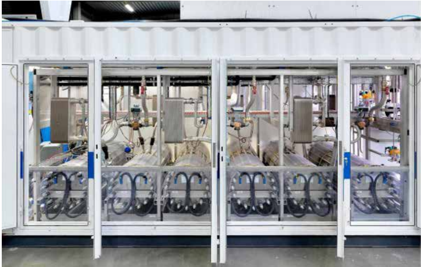
Hydrogen production of 90,000 liter/hour through electrolysis and integrated in a 20 ft sea container Photo courtesy of Hydrogenics Europe N.V.
